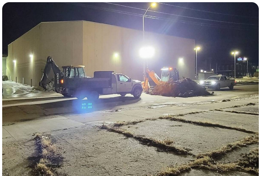
Ottumwa Water Works crews repairing a water main break.
