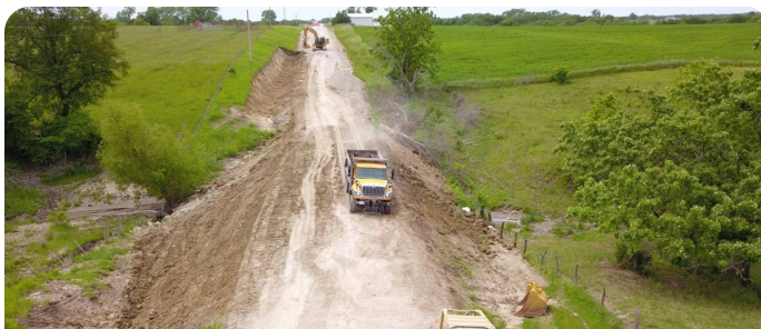
Rebuilding a damaged road and culvert: mitigation in action.
